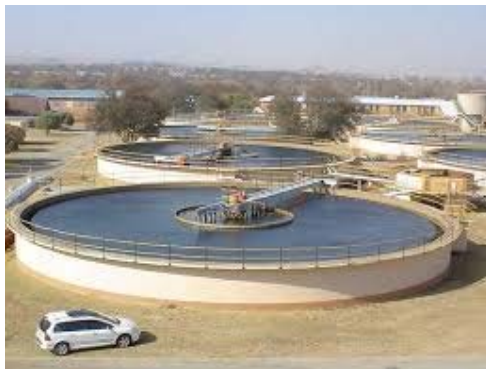
Picture 1. Midvaal water treatment plant in Klerksdorp.
