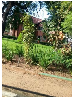
Administration block at block
