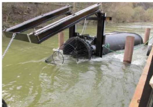
Figure 6. The River-Turbine prototype during installation. Source: KSB 2010. © KSB Aktiengesellschaft (2010)
